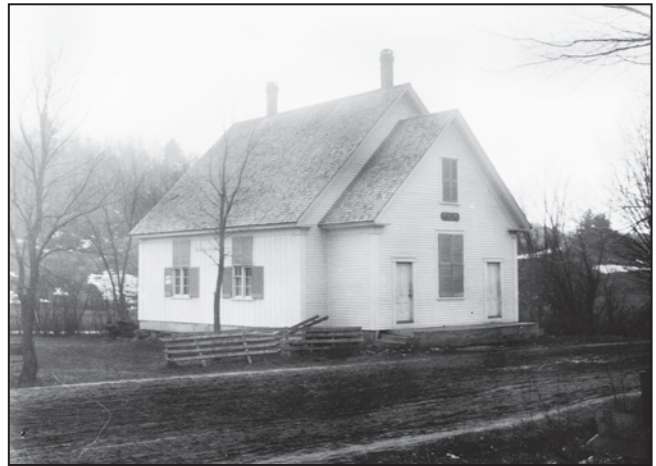
Original one-story Grange Hall, Mill Village, Goshen.
