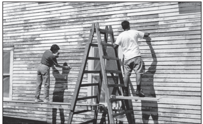
2003 repair of windows and exterior painting of Grange Hall.
