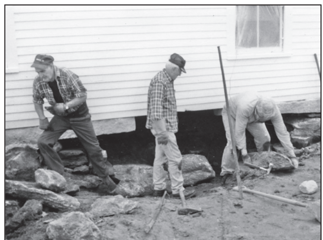
Volunteers repair the Grange Hall foundation, 2003.
